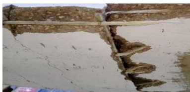
Fig. 12 Flexure–shear failure at mid-span of slab SHC
